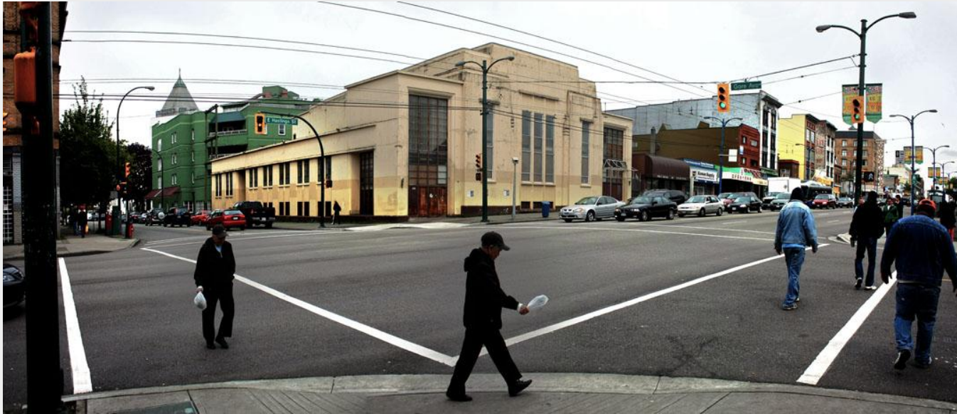
Figure 19: Hastings and Gore looking northeast.
