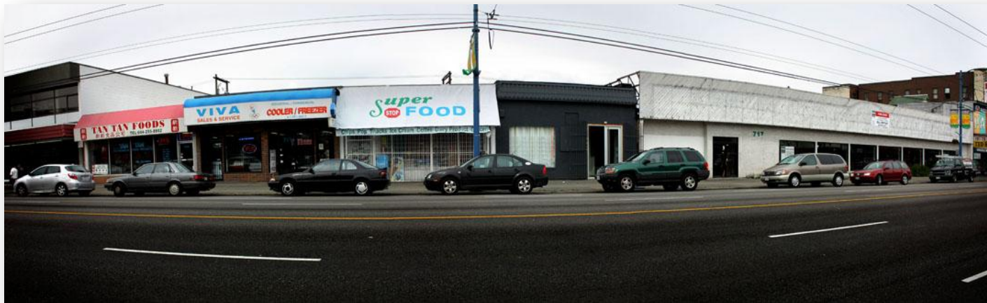
Figure 21: Hastings between Heatley and Hawks looking north.
