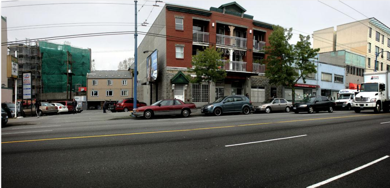
Figure 20: Hastings between Dunlevy and Jackson looking north/northeast.
